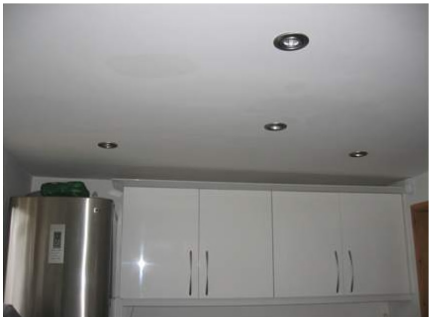
Ceiling Plastered and Decorated
